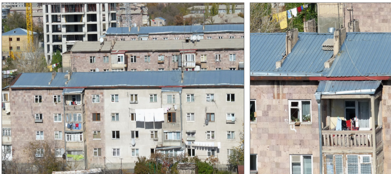
Image 10: Condominium in Yerevan – roofs repaired with sheet metal hoarding
