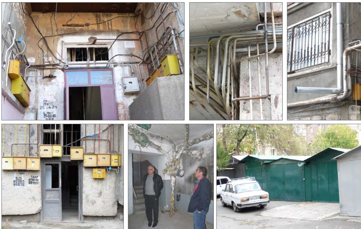
Image 8: Condominium in Yerevan – entrance areas, court yards, common space, simple repair works
