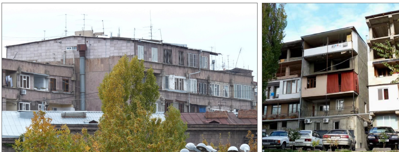
Image 11: Condominiums in Yerevan – construction of additional storeys
