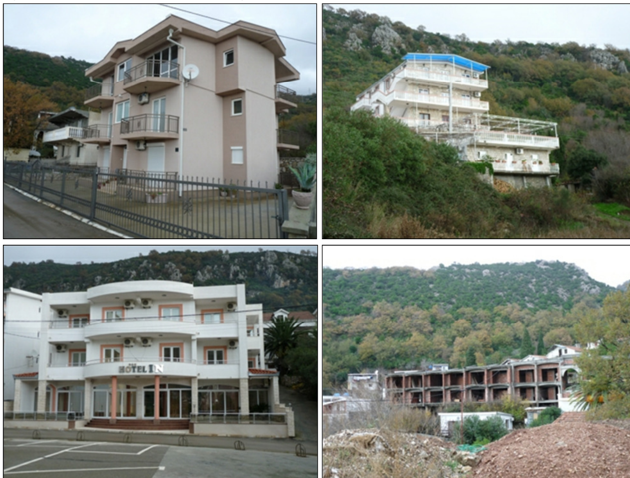
Figure 13: New informal hotels in Canj II
