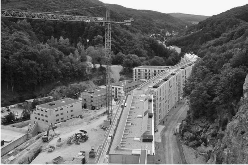
Figure 10.4b Waldmühle Rodaun: pictures of construction stages – difficult construction works.
