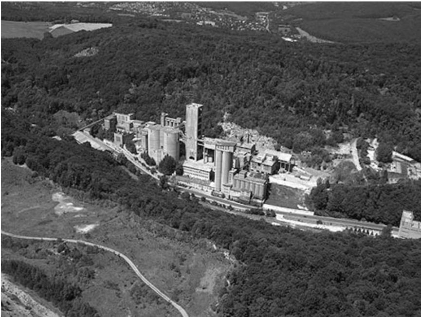
Figure 10.4a Waldmühle Rodaun: pictures of construction stages – cement factory before construction.
